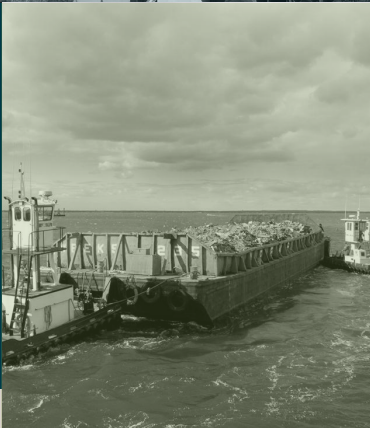
Debris Removal, Haul & Disposal Services
