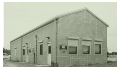
Mat Casting Yard
