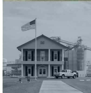
Lock Master Structure
