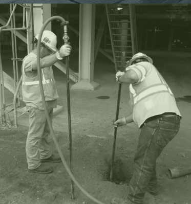
GPR, Utility Locating & Vacuum Excavation
